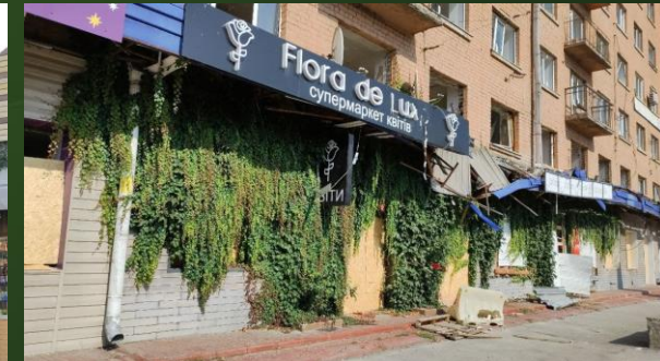
Surviving vertical greening damaged by a missile, Lukyanivka, Kyiv
